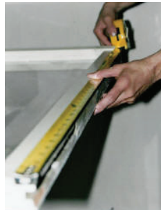
Figure 3. Measure the height of the upper sash.
