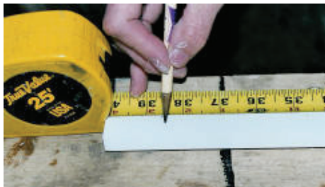
Figure 5. ...the top of Easy-Stop. Cut at the mark.
