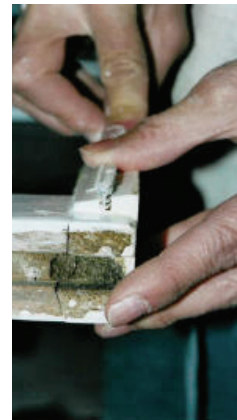
Figure 15 Install barbed-pile at meeting rail.
