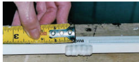
Figure 4. Transfer this measurement from the middle of the pile to...
