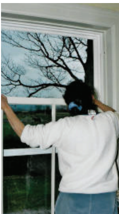
Figure 11. Attach ropes and install upper sash.
