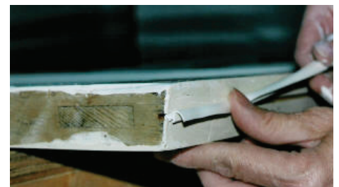
Figure 17. Install silicon flap on bottom.
