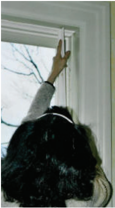
Figure 18. Install lower sash and interior stop.
