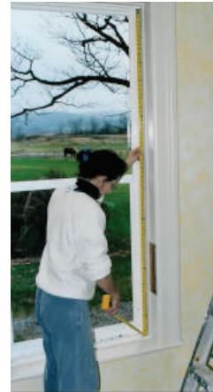
Figure 6. Measure the full height of the right side.
