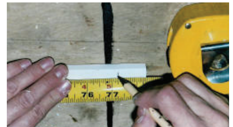
Figure 7. Mark and cut the bottom.
