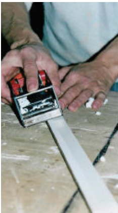
Figure 10. If necessary, plane for a snug fit. If loose, glue or nail in place.
