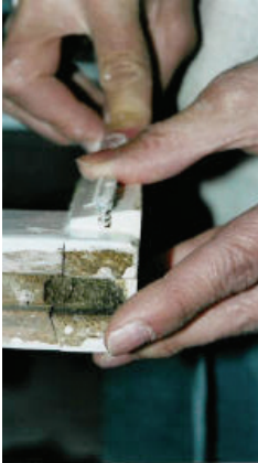
Figure 18. Install barbed-pile at meeting rail.
