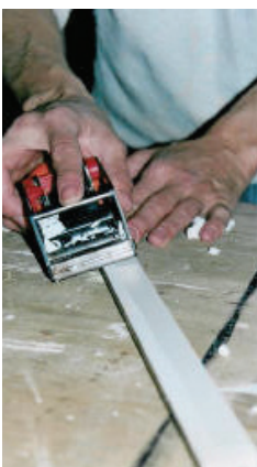
Figure 11. If necessary, plane for a snug fit. If loose, glue or nail in place.
