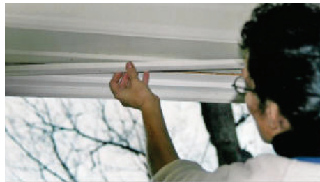
Figure 3. Cut and fit Easy-Stop head piece. Pile faces outwards.
