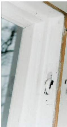
Figure 1. Begin by removing all existing parting-stops. (Aka parting-bead)
