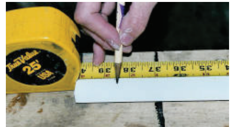
Figure 6. ...the top of Easy-Stop. Cut at the mark.
