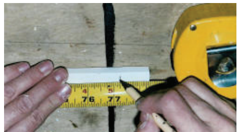
Figure 8. Mark and cut the bottom.
