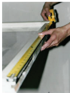
Figure 4. Measure the height of the upper sash.
