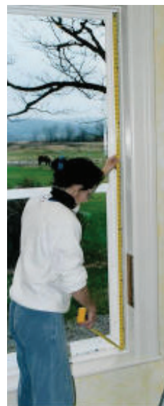
Figure 6. ...the top of Easy-Stop. Cut at the mark.
